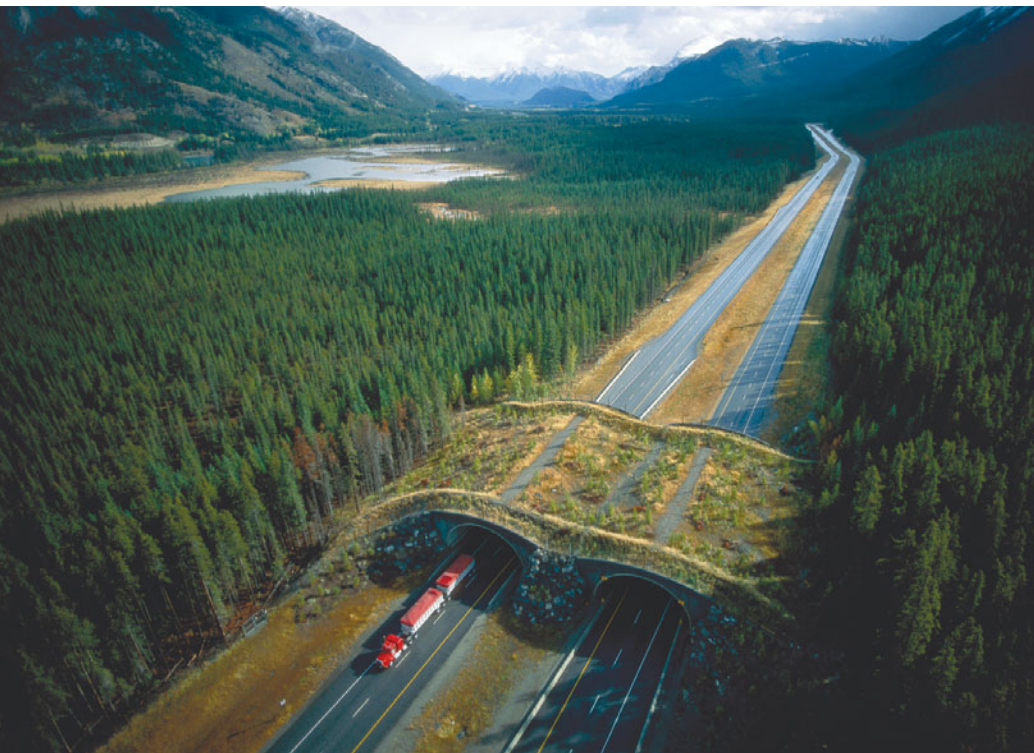
FIGURE 43.12 A Corridor for Large Mammals An overpass above the Trans Canada Highway in Banff National Park, Alberta. Bears, elk, deer and other large mammals use such overpasses, limiting the number of encounters with speeding vehicles that can have devastating effects for all involved.
